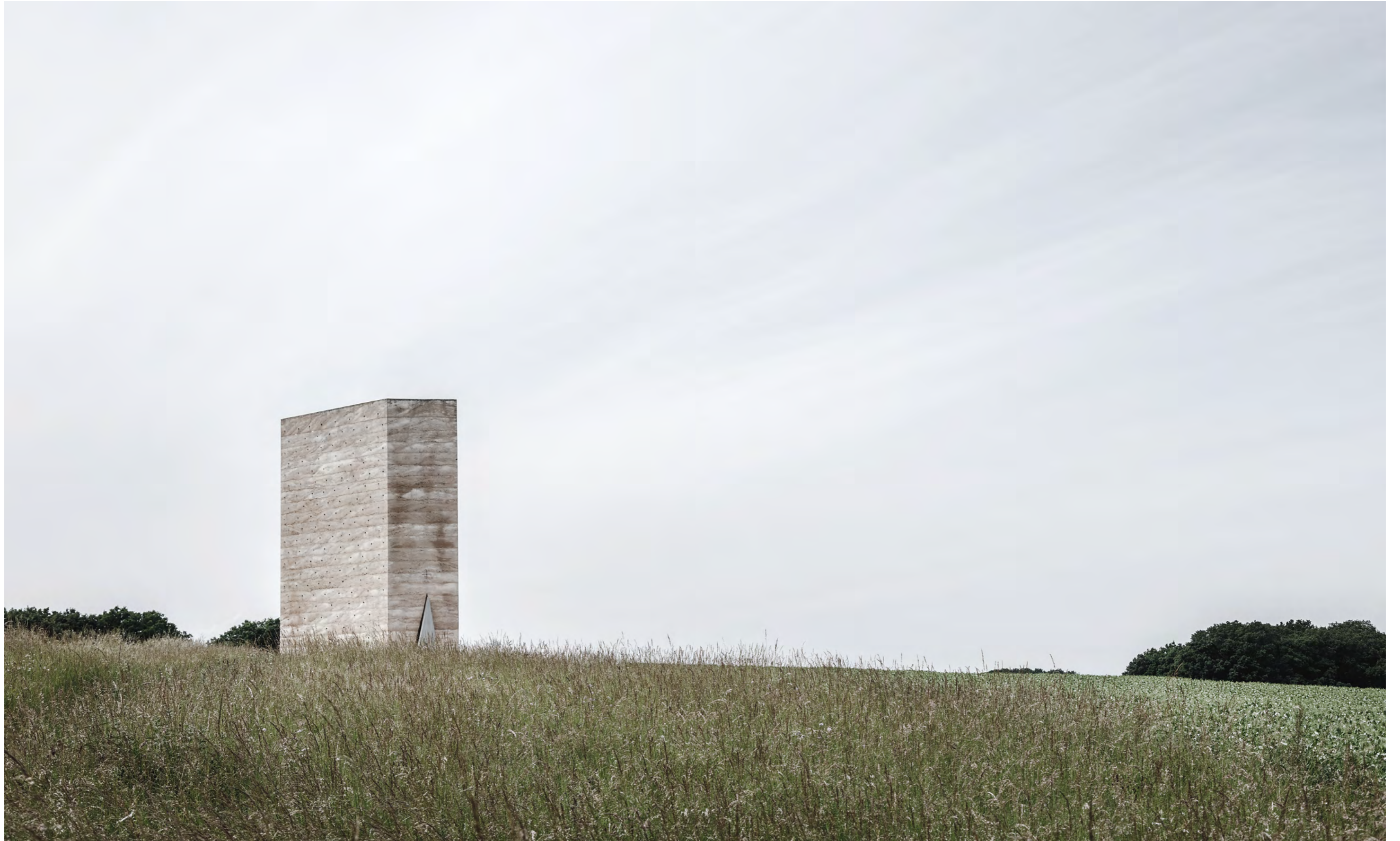
Bruder Klaus Field Chapel | Mechernich, Germany | 2007
